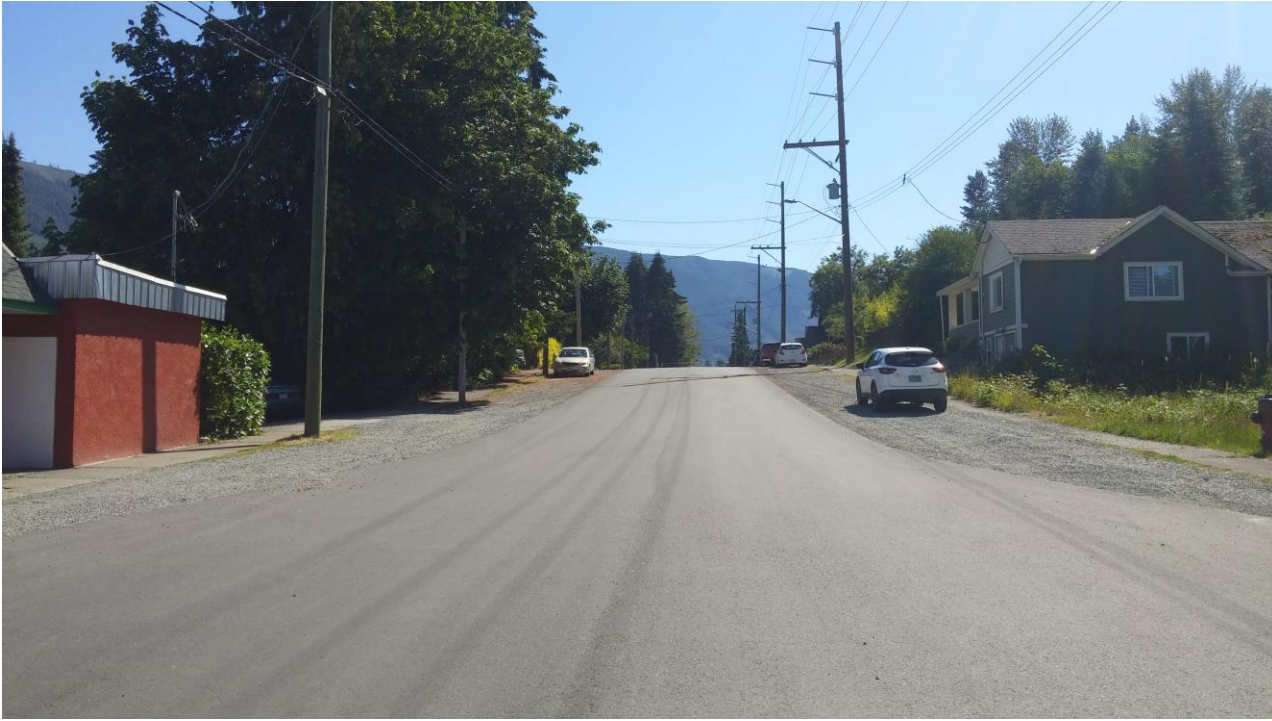
Cowichan Avenue street repaving
