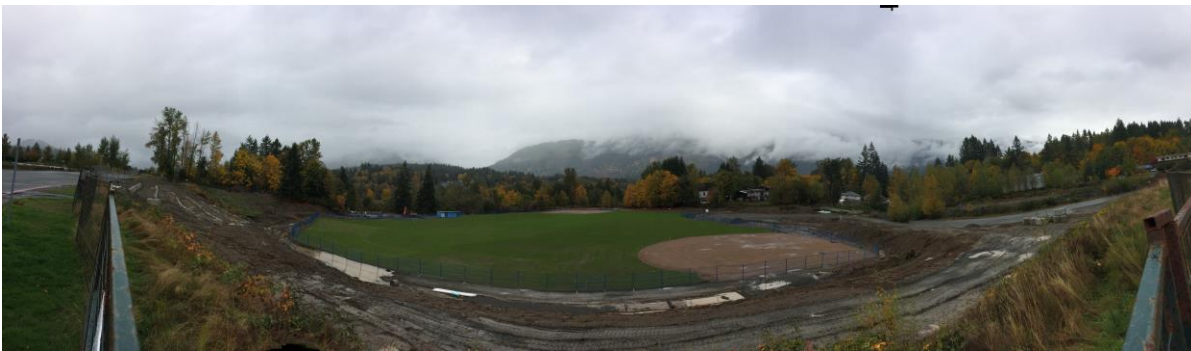
Centennial Park ballfields and soccer field at various stages of construction
