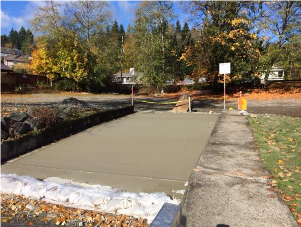
Boat launch repairs
